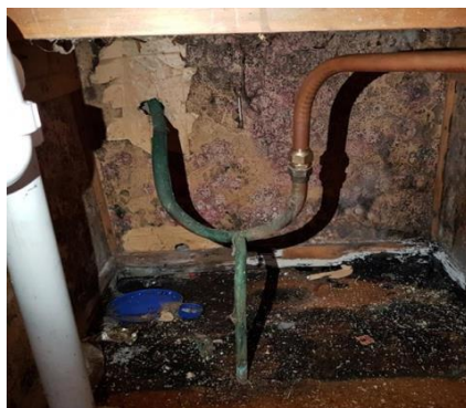
Hot water cupboards
