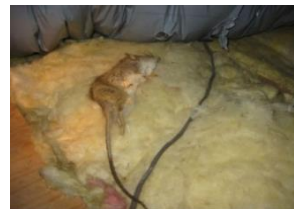
Wall and Ceiling Cavities
